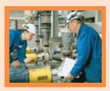
The efficiency of a Scottish wastewater pumping station has more than doubled since two AC drives were installed and interfaced with an ultrasonic level gauging system. This arrangement replaces simple on/off control of the motors, with the level monitored with a mechanical float
