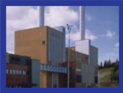
A peat power plant replaced inlet guide vanes with AC drives (total 300 kW) for its Primary air, Secondary air and Induced Draft fans. The electric power required to produce 1 MWh heat was reduced by 33% from 30 kWh to 20 kWh.
