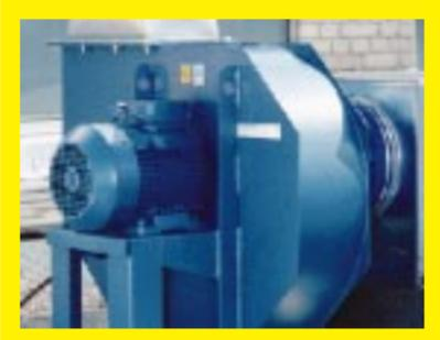
Dust is extracted from the flour milling process by 75 kW fans driven by electric motors. Fans were originally controlled by a star/delta starter, the motors running at full speed with airflow controlled by dampers. An AC drive was installed to control the fan speed.
