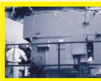
A Mexican iron mining company installed an AC drive, replacing the existing constant speed 1,250 kW cooling fan motor. Energy savings of 23% was achieved.
